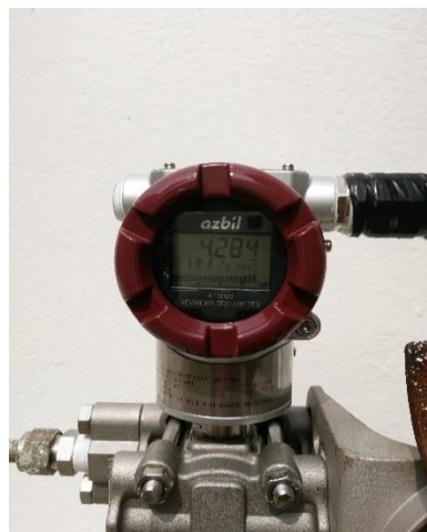
Gambar 3.15 DP Transmitter 4201 F
