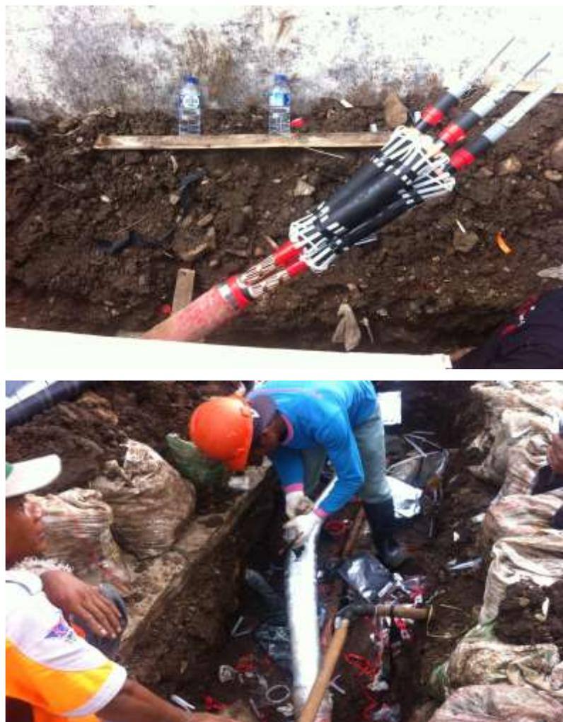
Gambar 3.2.2. Jointing Kabel
